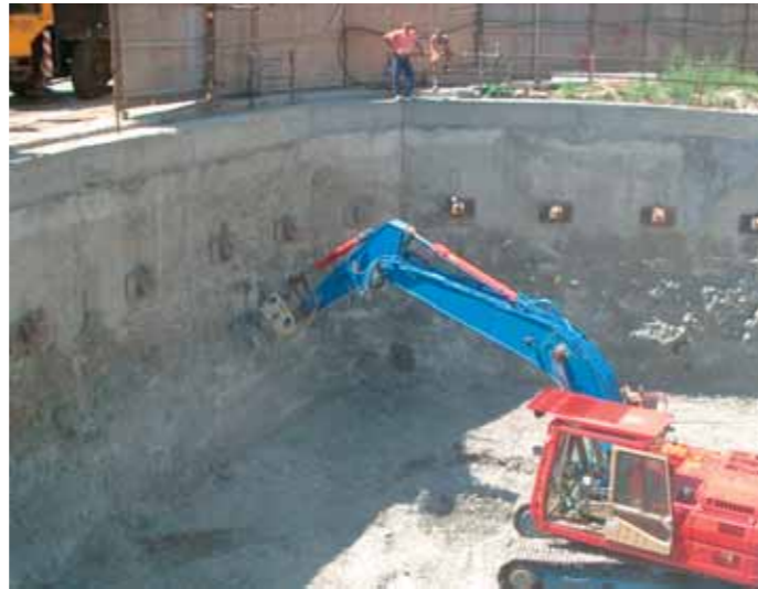
Demolitions and rough wall profiling, even with bracing, without damage to adjoining buildings.
